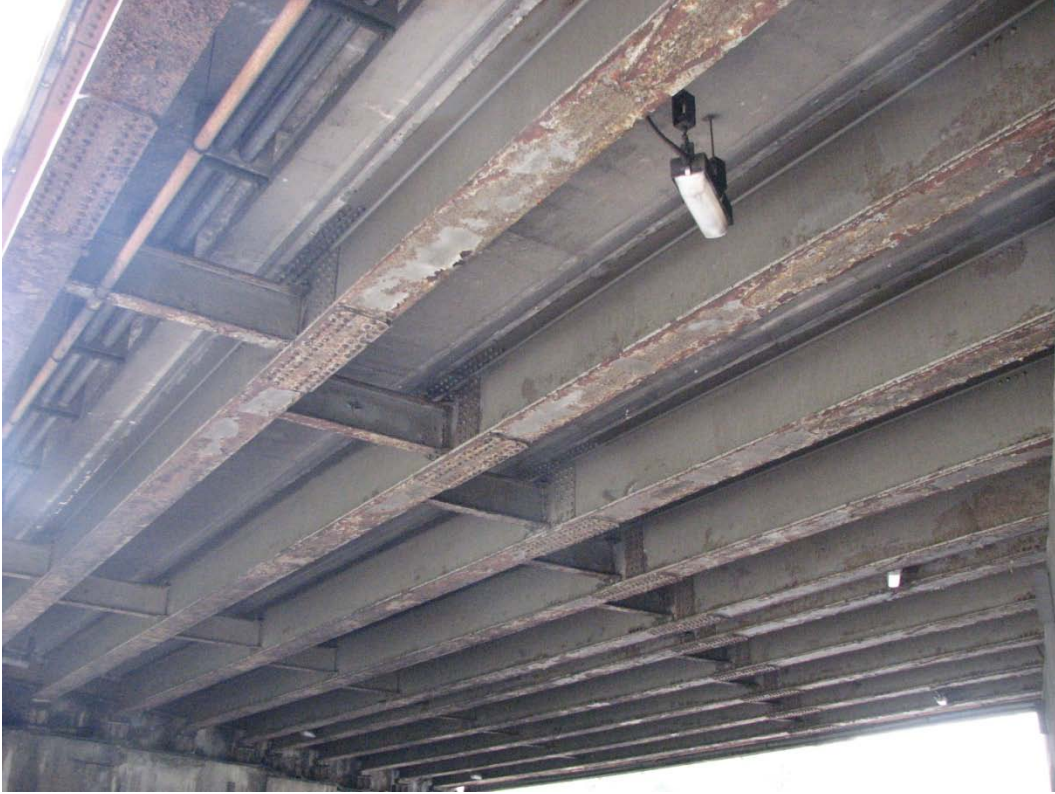
Photo 5 – Typical Underdeck Layout
