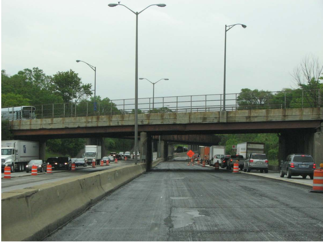
Photo 1 - Overall Looking West
