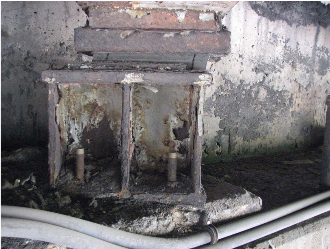
Photo 8 – Bearing Condition with Utilities
