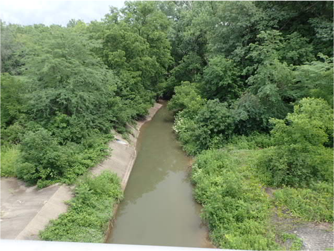
Photo 9 Channel Looking Upstream
