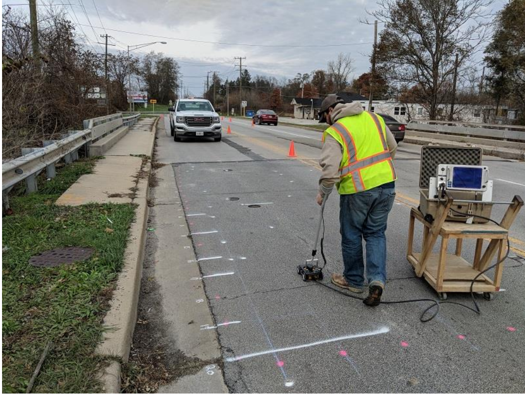
Photo 1) Performing GPR scan on 18" x18" grid pattern. (November 14, 2017)
