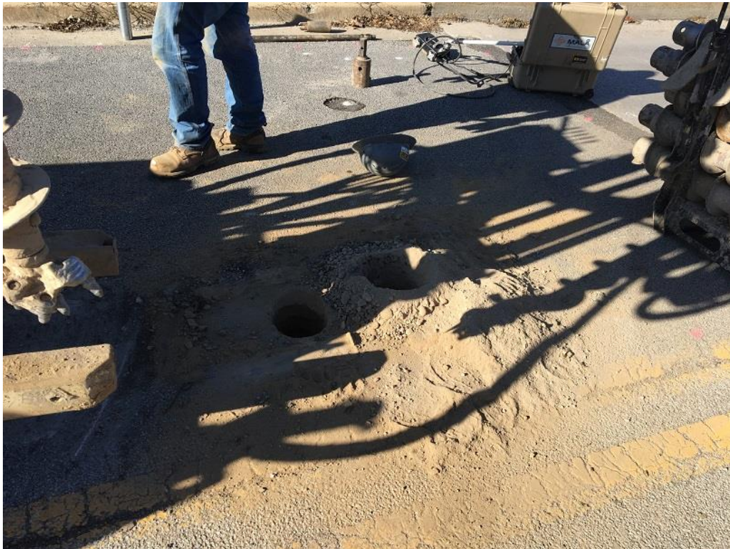
Photo 2) Overview of attempts #5 and #6 utilizing GPR data. Both holes encountered shallow obstructions. (November 20, 2017)
