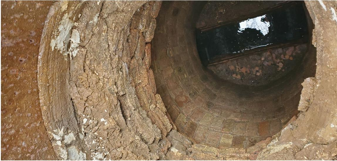
Existing Reconstructed San MH with precast cone section for reference (san mh sta 145+25 )
