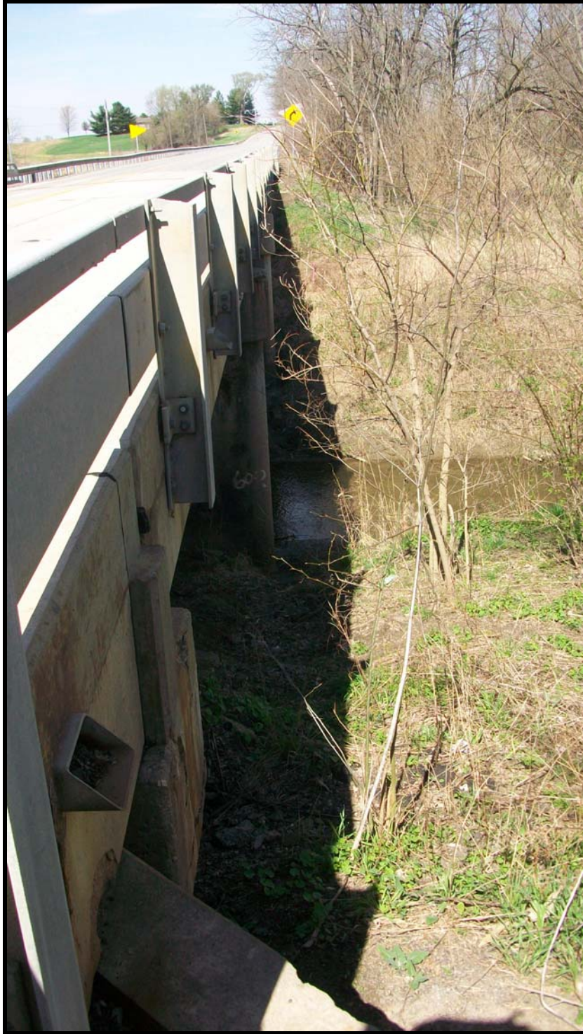
Photo 6- East Side of Bridge
