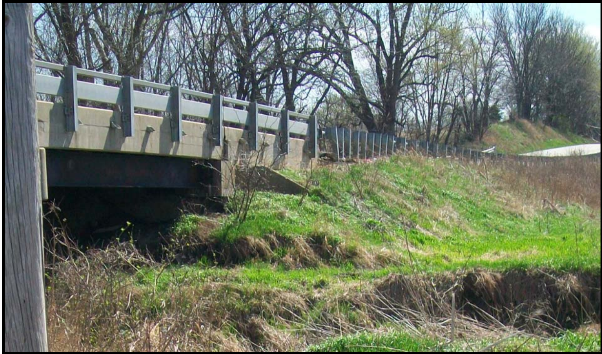
Photo 3- Southwest Corner of Bridge
