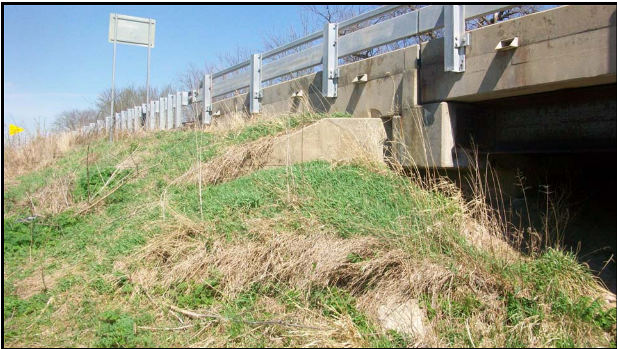
Photo 2- Northwest Corner of Bridge
