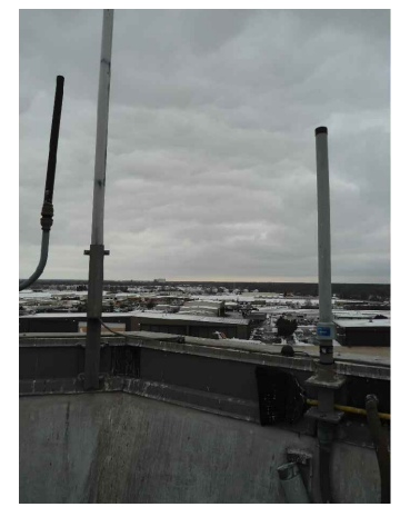
VIEW FROM WIRELESS ANTENNA TOWARDS ADS-B SITE
