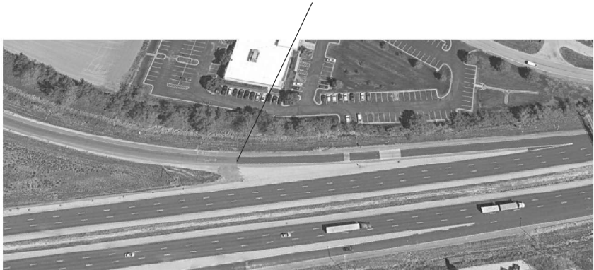
MICROSURFACING LIMITS WB 55/70 (RAMP 4, RAMP 1)
