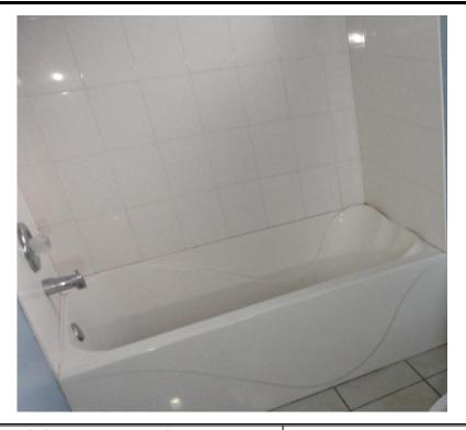
Material Description: Suspect ACM 8"X8" White Ceramic Tile Grout & Mortar
