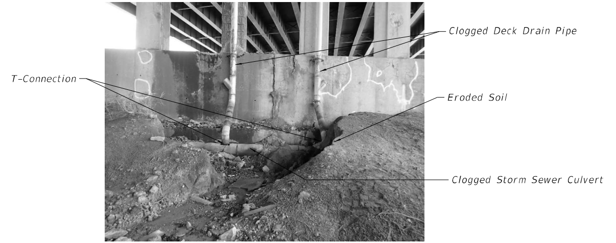
ELEVATION OF PIER 9 DRAINAGE SYSTEM
