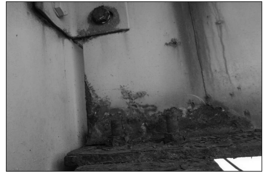
West Face of Stringer 1 at South Face of Floor Beam FB3
