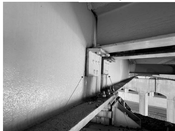
R8 Picture 12: P2; Beam 12 Looking E R14
