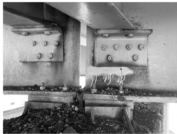
Picture 3: P2; Beam 6 Looking W R2
