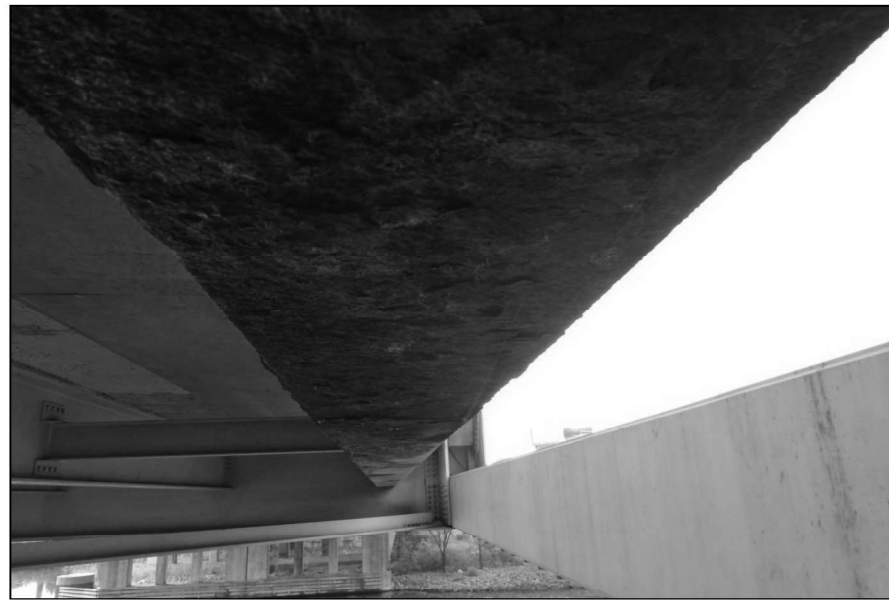
Bottom of Stringer 1 between Floor Beams FB3 and FB4 Looking South
