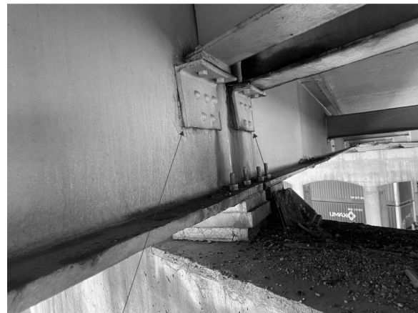
R12 Picture 20: P2; Beam 16 Looking E R18
