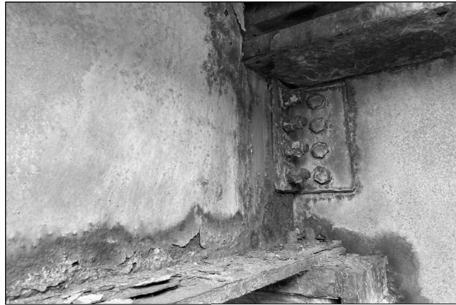
East Face of Stringer 8 at South Face of Floor Beam FB6
