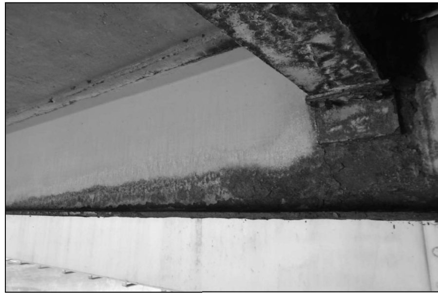
East Face of Stringer 1 at Floor Beam FB3 South Looking South
