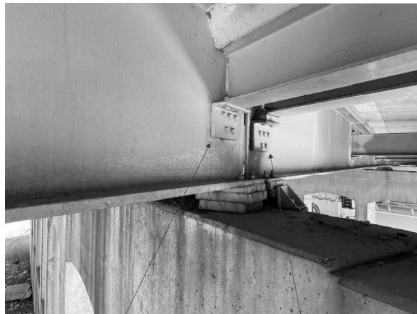
R1 Picture 2: P2; Beam 5 Looking E R5
