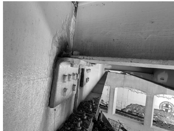
R2 Picture 4: P2; Beam 6 West Face
