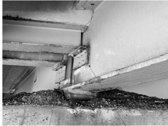
R16 Picture 17: P2; Beam 14 Looking W R10
