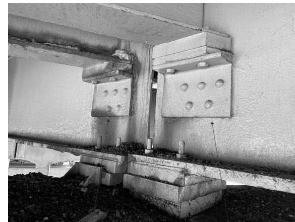
R15 Picture 15: P2; Beam 13 Looking W R9
