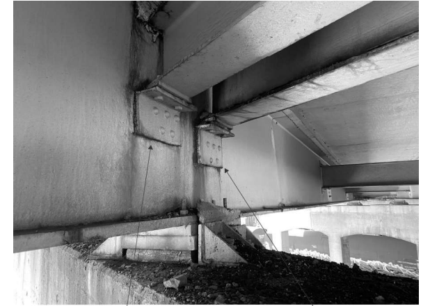
R13 Picture 23: P2; Beam 17 Looking E R19
