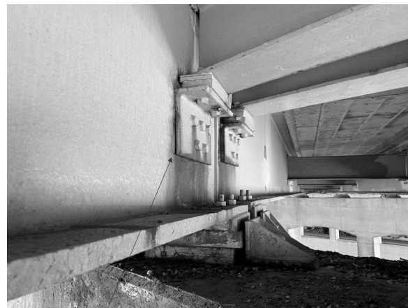
R4 Picture 11: P2; Beam 9 Looking E
