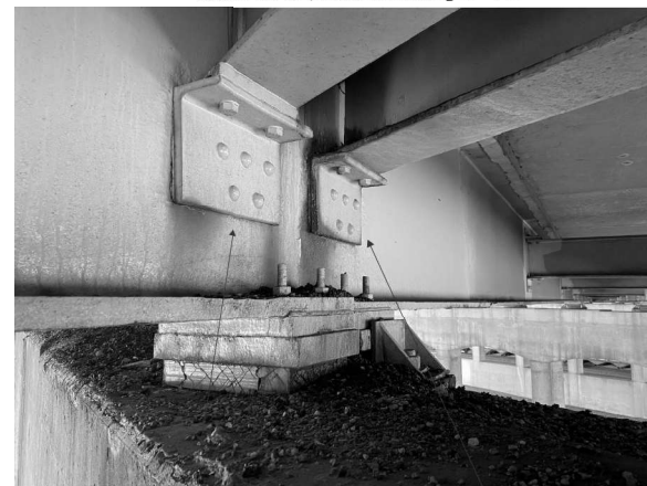
R9 Picture 14: P2; Beam 13 Looking E R15
