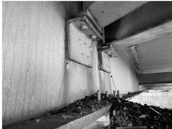
R11 Picture 18: P2; Beam 15 Looking E R17
