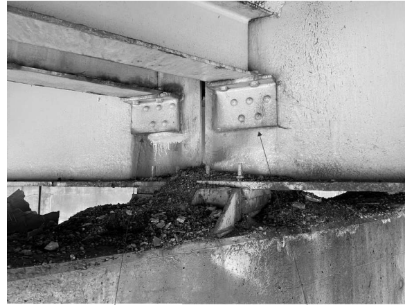
R17 Picture 19: P2; Beam 15 Looking W R11
