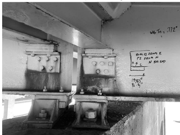
Picture 10: P2; Beam 9 Looking W R4
