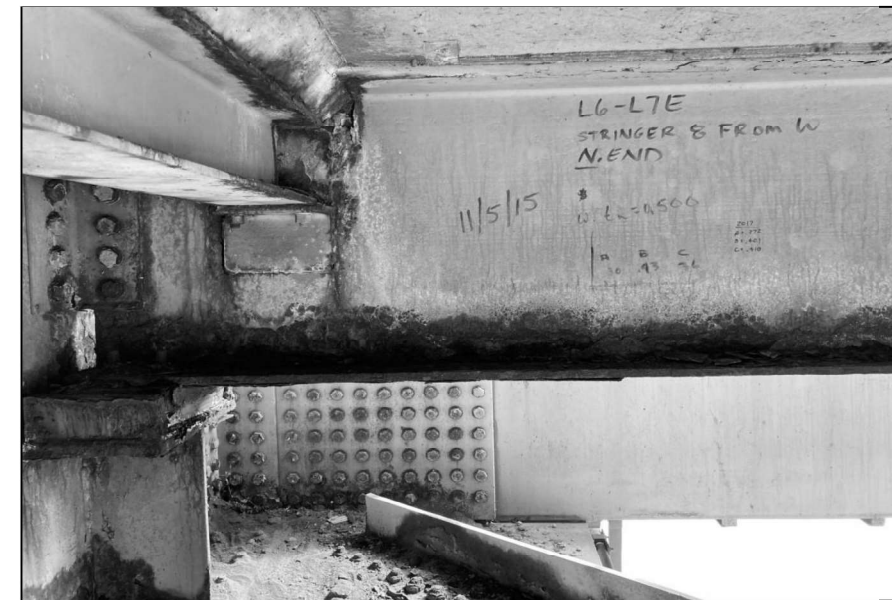
West Face of Stringer 8 at South Face of Floor Beam FB6
