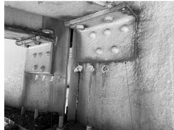
R19 Picture 22: P2; Beam 17 Looking W R13
