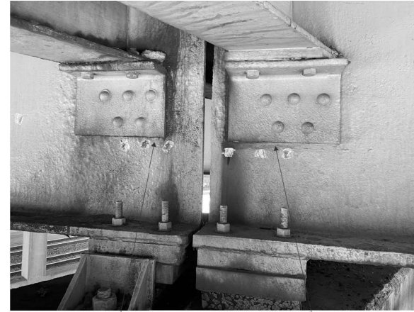
R18 Picture 21: P2; Beam 16 Looking W R12
