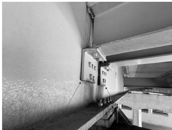
R3 Picture 9: P2; Beam 8 Looking E R7
