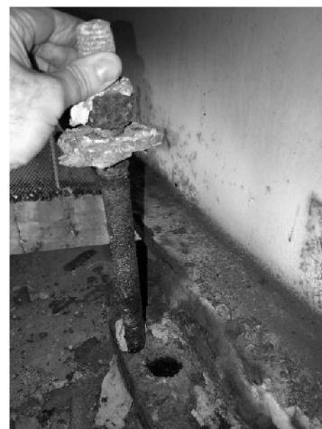
PHOTO 1: REPAIR ANCHOR BOLT
