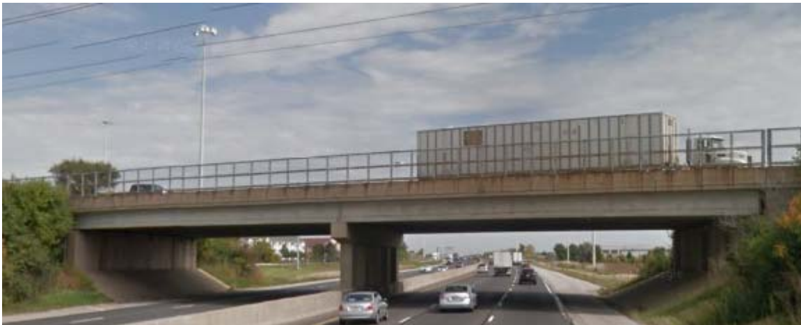
Exhibit 2 Weber Road over I-55 (southbound on I-55)
