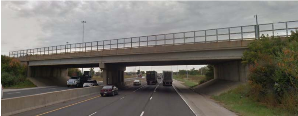
Exhibit 3 Weber Road over I-55 (northbound on I-55)
