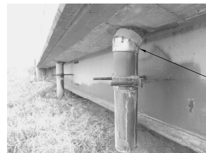
*DRAIN DOWNSPOUT IMAGE
