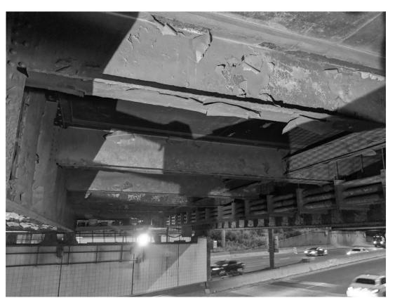
Photo 3: West Span, Typical Diaphragms, looking east
