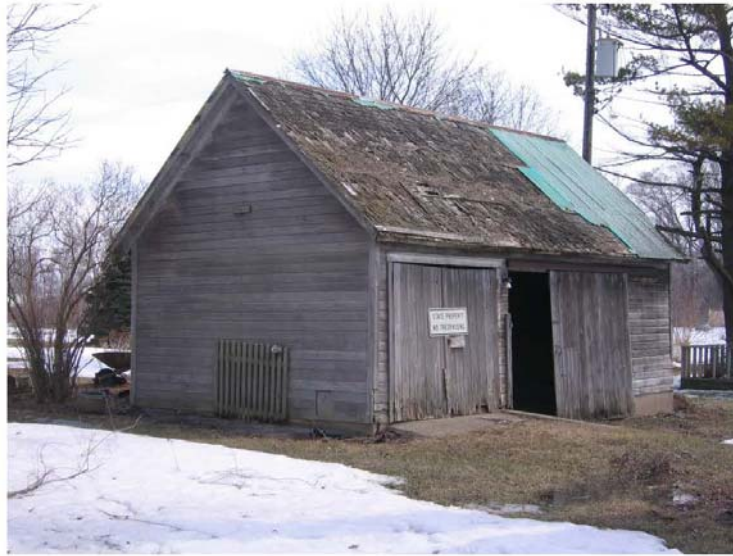
Shed North Face
