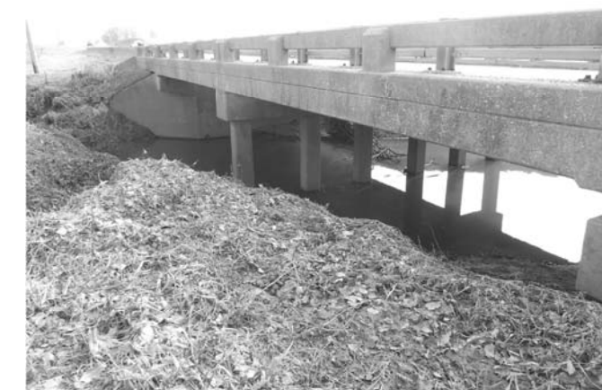
ELEVATION VIEW ⑦ (Looking Southwest)
