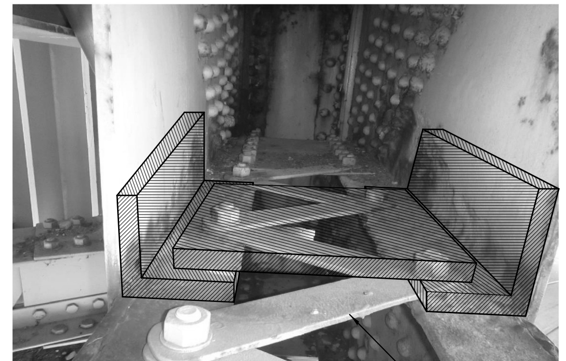
BENT R REPAIR DETAILS
