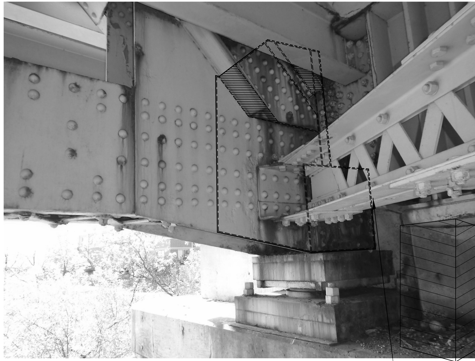
PHOTO - EAST TRUSS (L0) WEST GUSSET - LOOKING EAST
