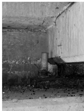
EXISTING BOLT AT NORTH ABUTMENT
