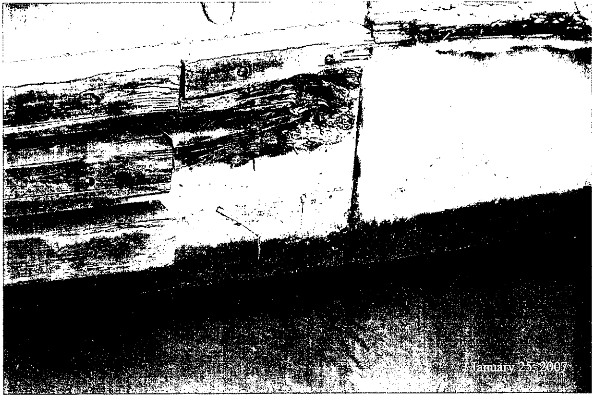
Damaged and missing timbers at nouth corner of west abutment
