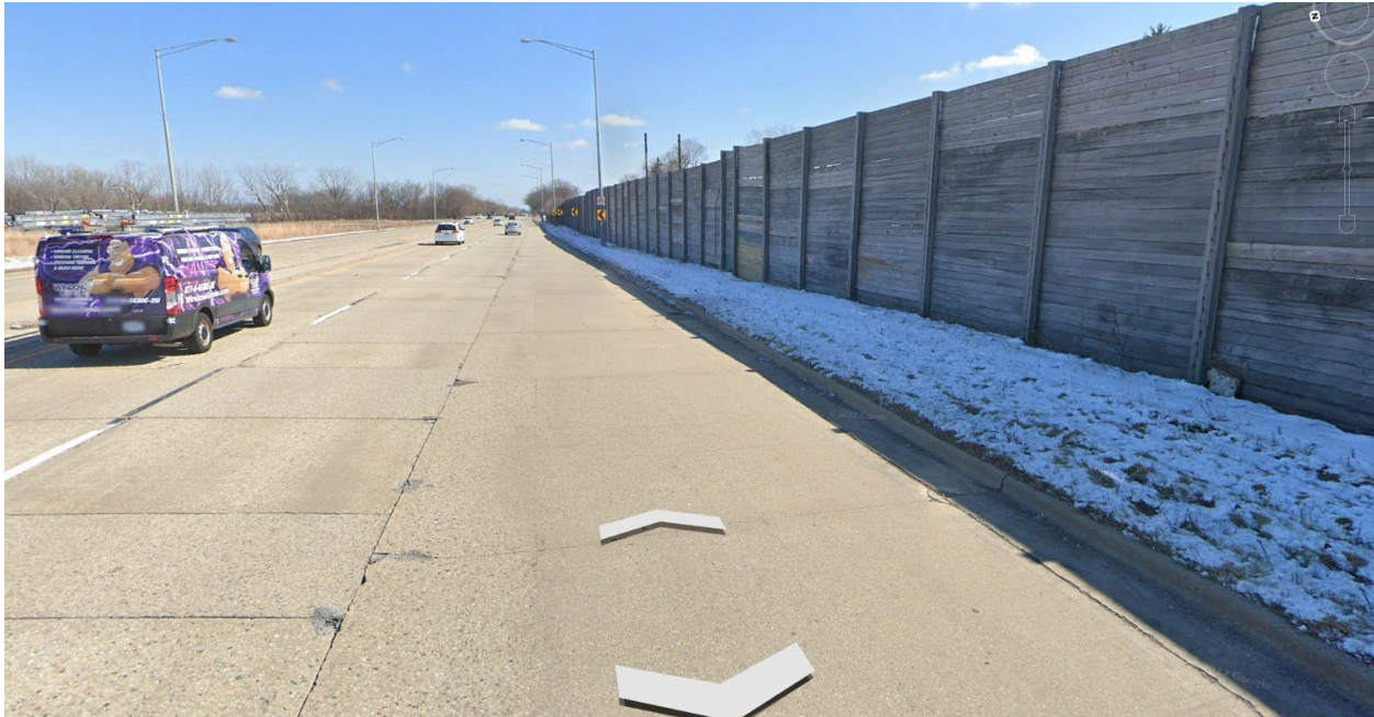
Exhibit 2d – Existing Site Conditions, Looking East along EB Lake Cook Road at the East Wall
