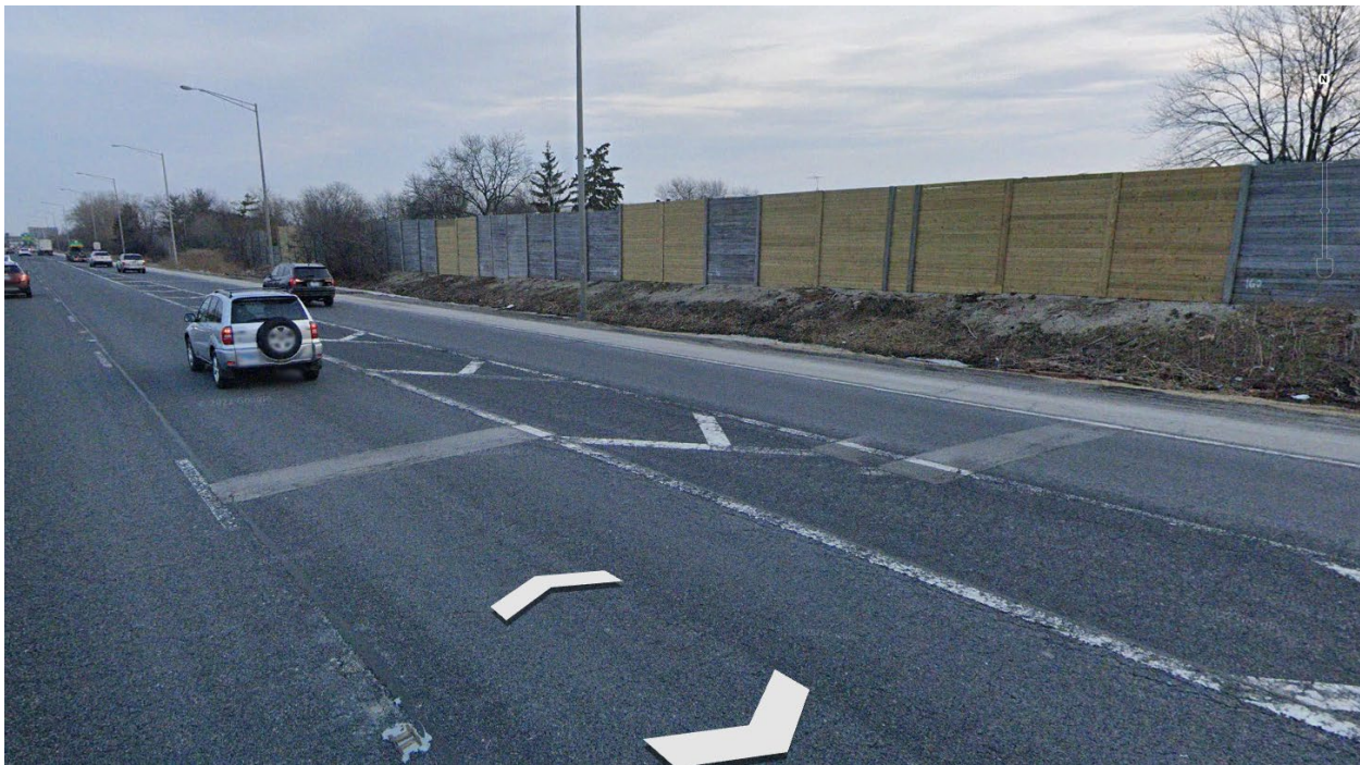
Exhibit 2a – Existing Site Conditions, Looking South along SB IL 53 at the West Wall
