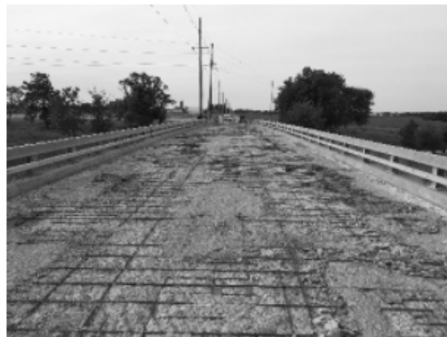
PHOTOGRAPH NO. 1 (Showing general condition of existing deck.)
