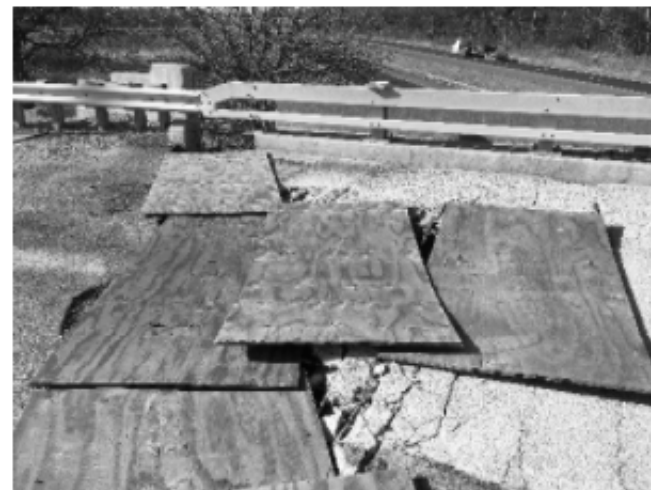
PHOTOGRAPH NO. 2 (Showing plywood covering holes in existing deck.)
