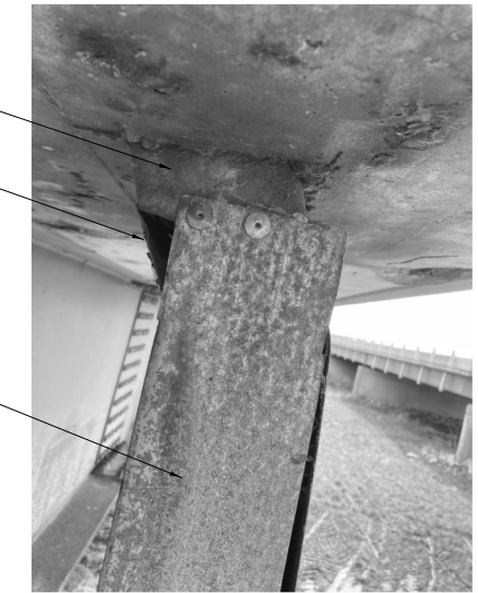
EXISTING DECK DRAIN TO DRAIN EXTENSION JUNCTION (TYP.)
