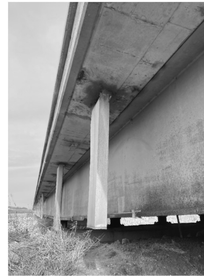
EXISTING DECK DRAIN EXTENSION (TYP.)
