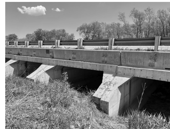
REMOVE EXISTING RAILING - WEST END OF CULVERT
