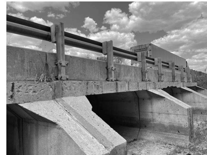
REMOVE EXISTING RAILING - EAST END OF CULVERT
