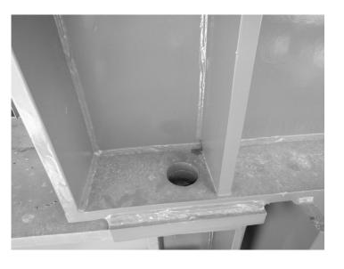
PHOTO 2 (Showing missing bolt)
