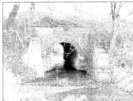
Stone Masonry Arch Structure (Looking North/Downstream)
