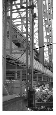
■Replace Each Span Navigation Light Assembly with LED Navigation Light Assemblies at Exisiting Mounting Brackets
