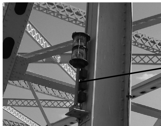
EXISTING WHITE NAVIGATION LIGHT (TYPICAL)
