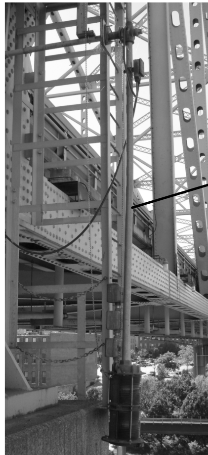
EXISTING NAVIGATION LIGHT (TYPICAL)
