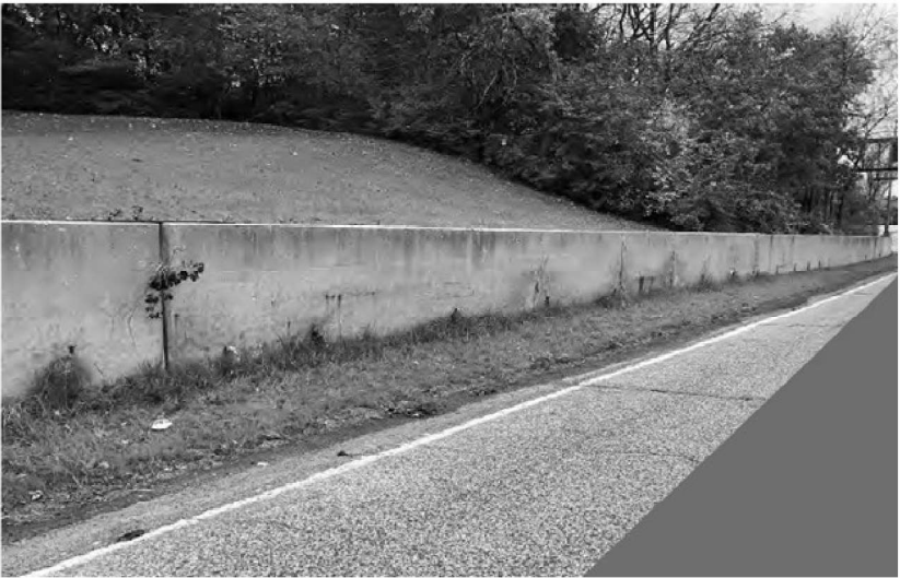
PARTIAL VIEW OF EXISTING WALL
