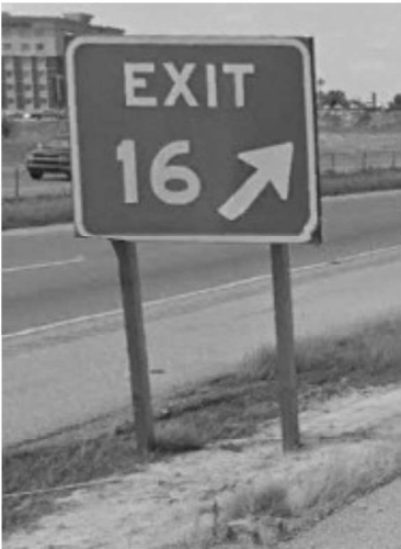
SIGN NO. EX034 STA 772+64.00, LT WEST BOUND
