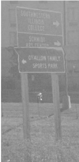
SIGN NO. EX121 STA 18+67.00, RT RAMP A
