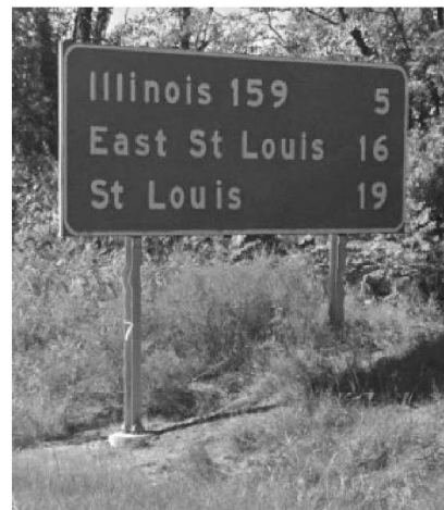
SIGN NO. EX061 STA 850+00.00, LT WEST BOUND
