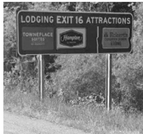
SIGN NO. EX062 STA 858+58.00, LT WEST BOUND
