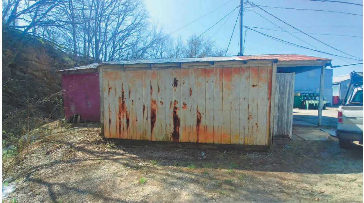
Old Maintenance - North Face
