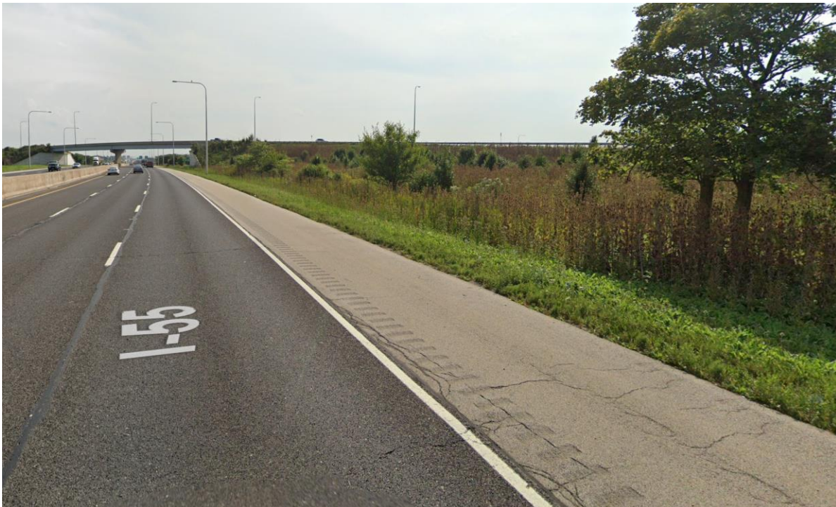
Exhibit 2 – Existing Site Conditions at Proposed Wall Location, Looking south along I-55 SB
