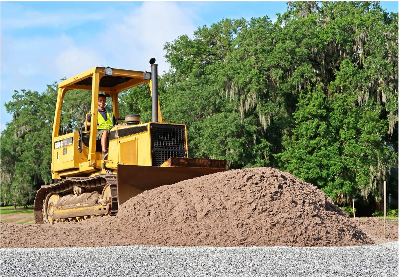
**THE ROOTZONE MIXTURE SHOULD BE SPREAD AND UNIFORMLY FIRMED TO A 12-INCH DEPTH WITH A TOLERANCE OF PLUS OR MINUS 1 INCH.**
