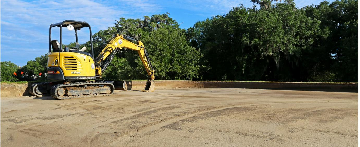
**THE SUBGRADE MUST BE SMOOTH, FIRMLY COMPACTED AND FREE OF WATER-COLLECTING DEPRESSIONS.**
