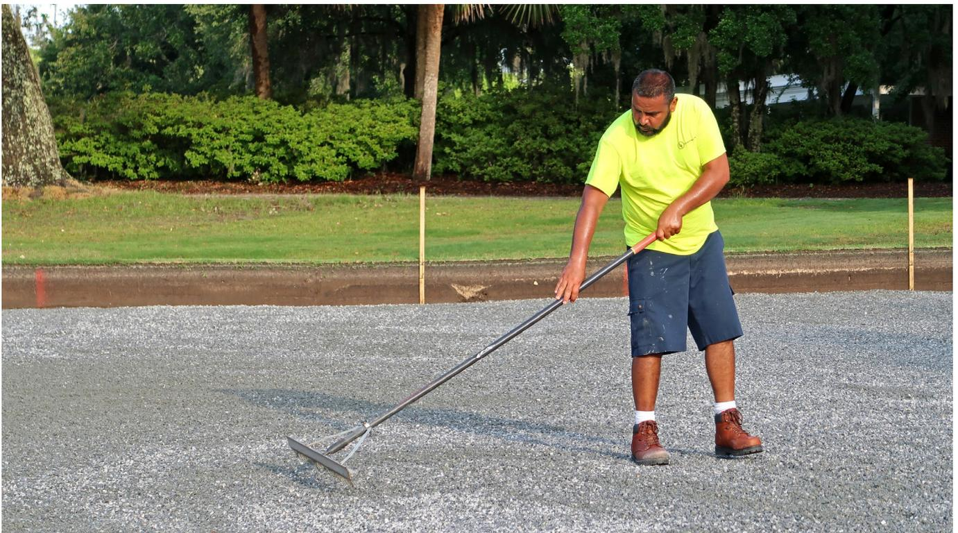
**THE GRAVEL LAYER SHOULD BE SPREAD TO A MINIMUM DEPTH OF 4 INCHES AND SHOULD MIRROR THE FINAL SURFACE OF THE PUTTING GREEN.**
