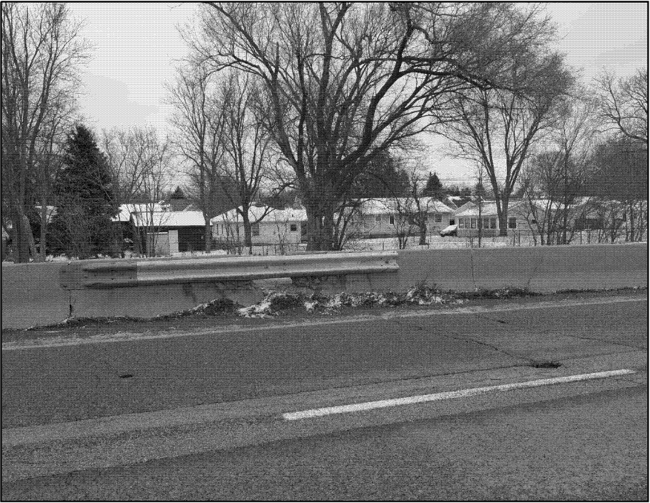
LOCATION 13 US-20 APPX. 0.3 MILES WEST OF IL-31 REPLACE 14 FT OF MEDIAN BARRIER WALL
