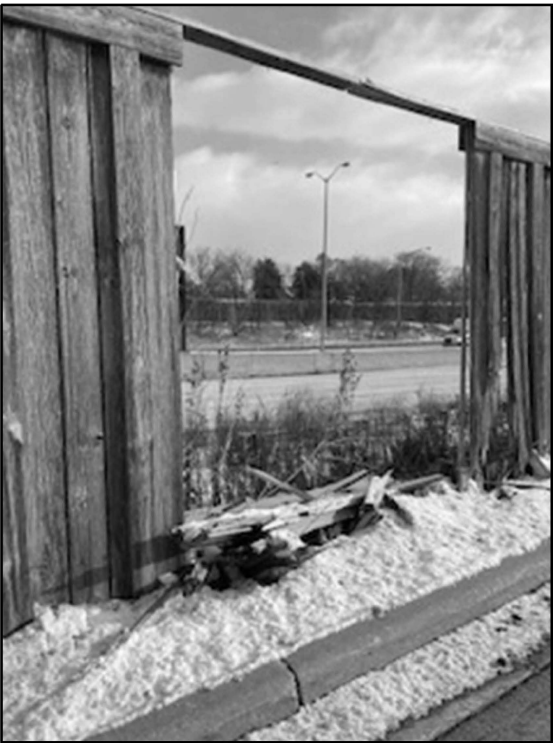
LOCATION 30 I-290 EB ABOUT 0.15 MILES EAST OF EMROY AVE. REPLACE ONE SECTION 12' X 10' WOOD NOISE WALL
