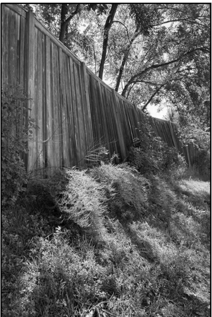
LOCATION 25 IL-83 NB ABOUT 0.30 MILES SOUTH OF US-34 (OGDEN AVE.) REPLACE EIGHT SECTIONS 9' X 12' EACH WOOD NOISE WALL WITH POSTS
