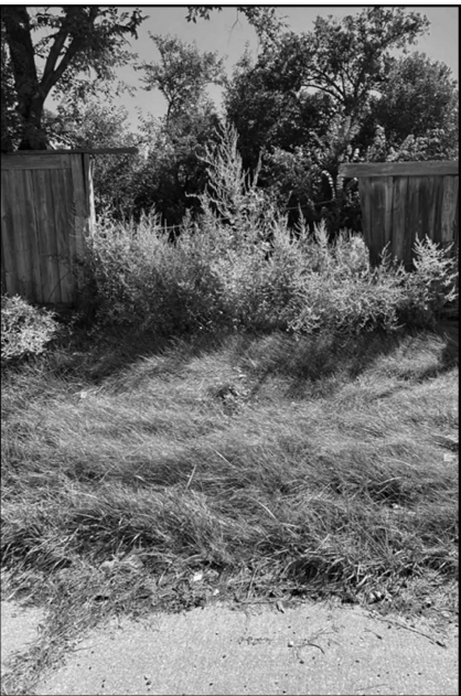
LOCATION 24 IL-83 NB ABOUT 0.17 MILES SOUTH OF US-34 (OGDEN AVE.) REPLACE TWO SECTIONS 9' X 6' EACH WOOD NOISE WALL WITH POSTS
