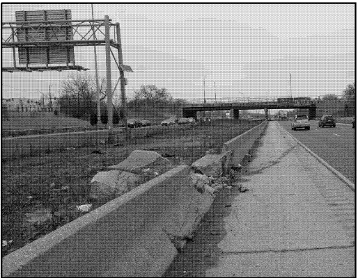
LOCATION 6 I-94 NB MEDIAN ABOUT 0.10 MILES WEST OF MARTIN LUTHER KING DR. REPLACE 23 FT OF SHOULDER BARRIER WALL
