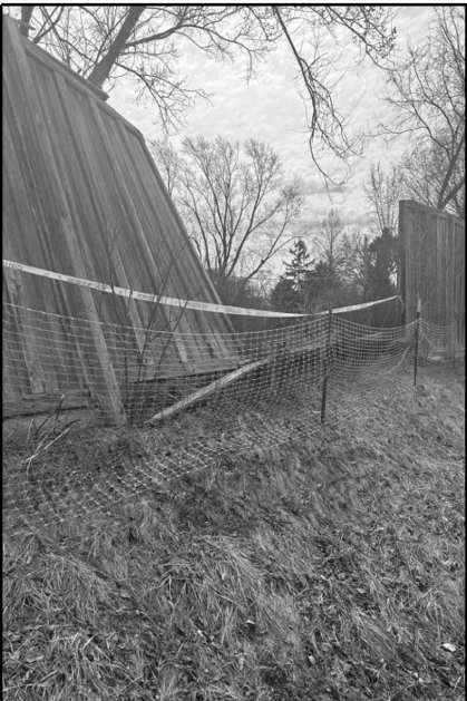
LOCATION 26 IL-83 NB ABOUT 0.35 MILES NORTH OF US-34 (OGDEN AVE.) REPLACE EIGHT SECTIONS 8' X 12' EACH WOOD NOISE WALL WITH POSTS
