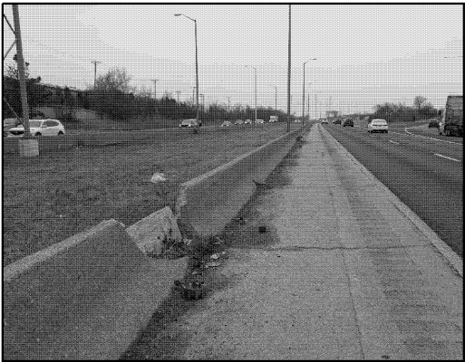
LOCATION 9 I-94 SB ABOUT 130' EAST OF COTTAGE GROVE REPLACE 8 FT OF SHOULDER BARRIER WALL
