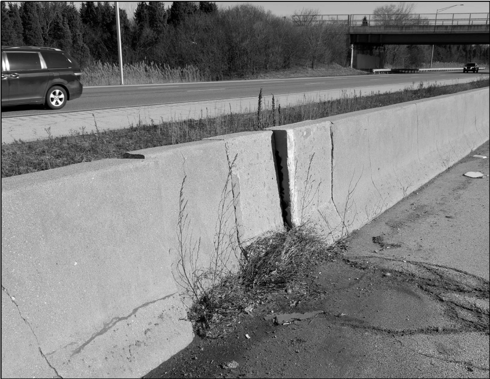
LOCATION 12 I-290 EB ABOUT 340' WEST OF MILL RD. REPLACE 4 FT OF SHOULDER BARRIER WALL
