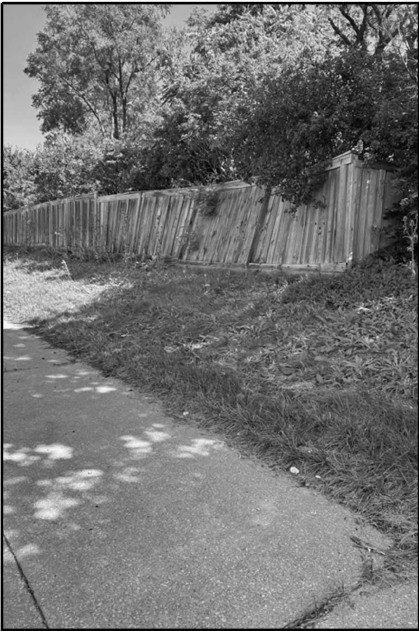
LOCATION 23 IL-83 NB ABOUT 0.15 MILES SOUTH OF US-34 (OGDEN AVE.) REPLACE THREE SECTIONS 9' X 6' EACH WOOD NOISE WALL WITH POSTS
