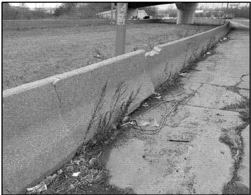
LOCATION 7 I-94 NB JUST SOUTH OF 100TH ST. REPLACE 23 FT OF SHOULDER BARRIER WALL
