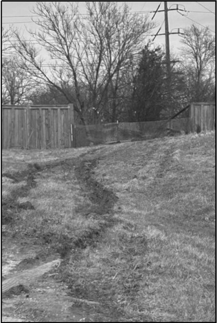
LOCATION 27 IL-83 NB NEAR BURLINGTON AVE./RAILROAD REPLACE FIVE SECTIONS 8' X 12' EACH WOOD NOISE WALL WITH POSTS
