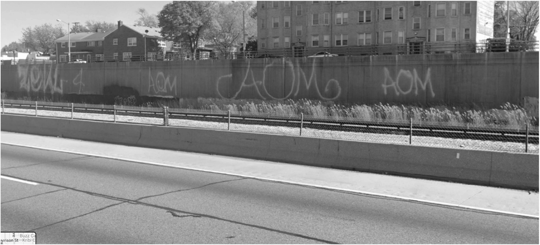
TYPICAL VIEW OF RETAINING WALL BETWEEN HOME AVE AND AUSTIN BLVD
