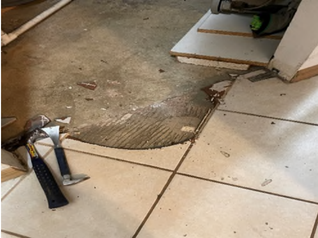
HA-6: 12" x 12" Gray Stone/Ceramic Floor Tile Thin Set and Mortar
