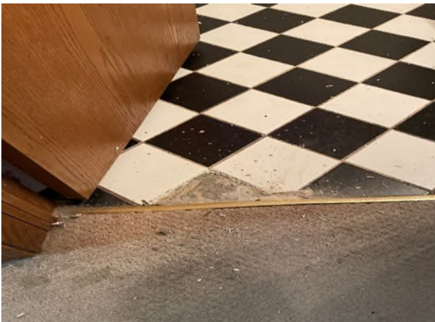
HA-8: 4" x 4" Black Stone/Ceramic Floor Tile Thin Set and Grout
