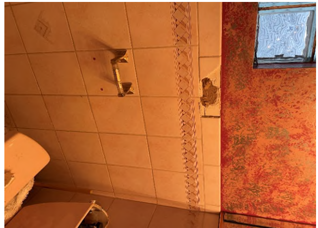
HA-9: 3" x 3" White Ceramic Wall Tile Mastic and Grout
