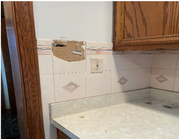
HA-2: 6" x 8" White Wall Tile Mastix and Grout
