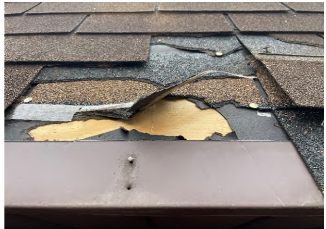
HA-9: Black Asphalt Roof Shingle HA-10: Black Tar/Felt Paper under HA-9
