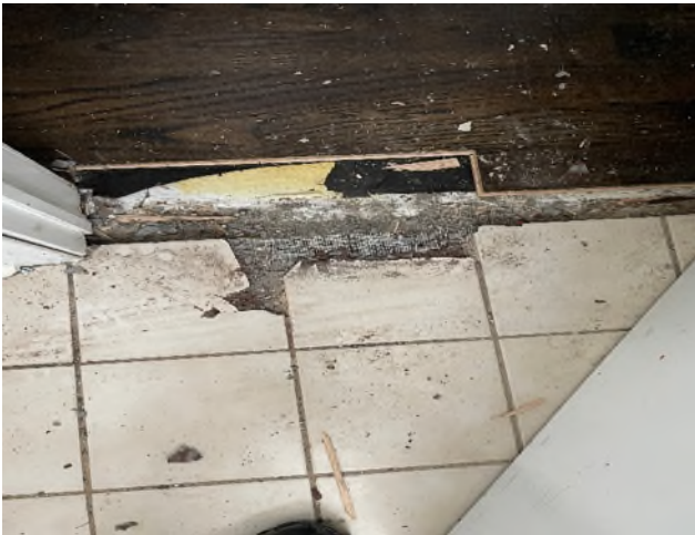
HA-2: White 8” x 8” Stone Floor Tile Grout and Thin Set
