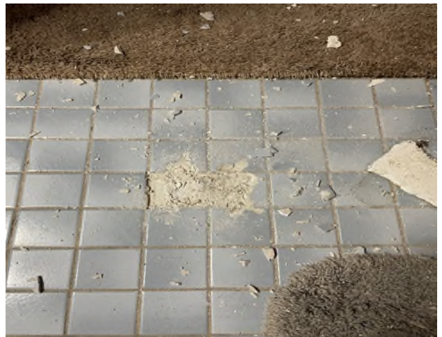
HA-3: Brown 2" x 2" Ceramic Floor Tile Thin Set and Grout
