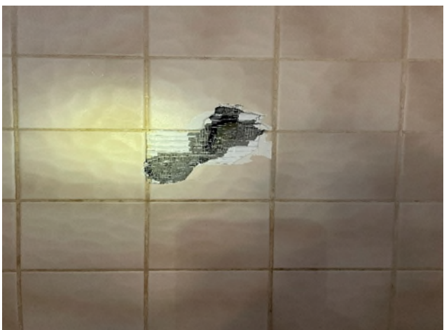
HA-4: Tan 8" x 8" Ceramic Wall Tile Mastic and Grout
