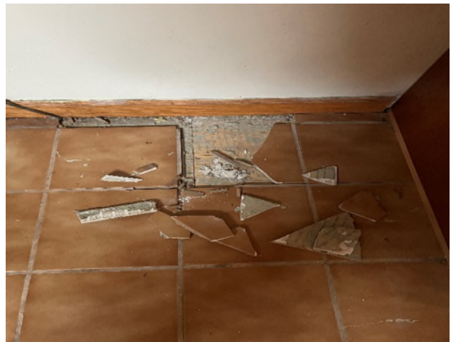
HA-1: 8" x 8" Tan Floor Tile Thin Set and Grout
