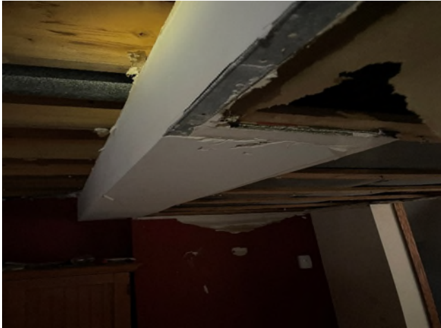
HA-7: White Wall/Ceiling Joint Compound HA-17: Gypsum Board
