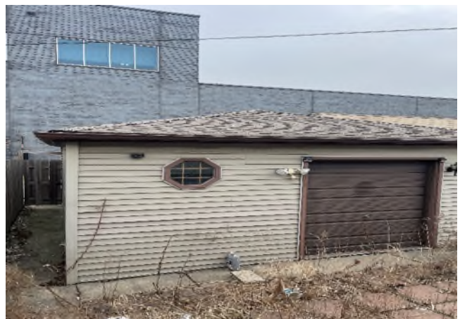
HA-13: Black Asphalt Shingle HA-14: Tar/Felt Paper under HA-13 HA-15: Black Tar Paper under Siding
