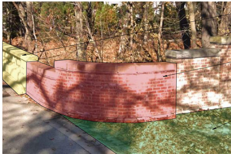
2 VIEW OF SE MASONRY WALL - LOCATION 2
