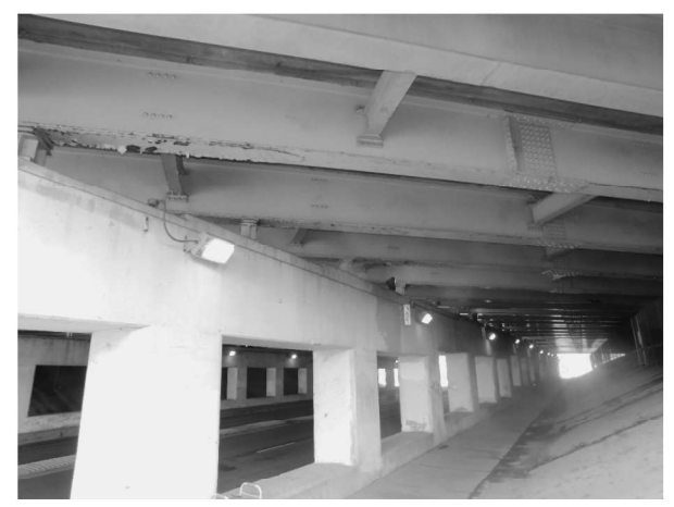
EXISTING LIGHTING: PIER 1 (Looking South)
