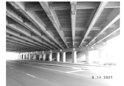
EXISTING LIGHTING: PIER 2 (Looking North)
