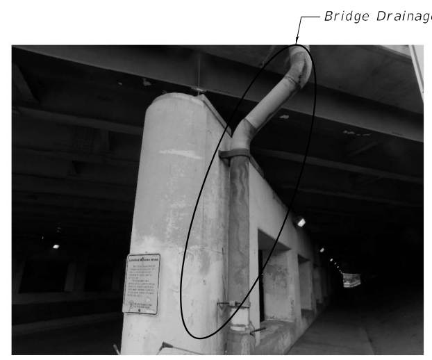
EXIST. DRAINAGE SYSTEM REPAIR: LOCATION 1 - PIER 1 (Looking South)
