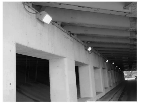
EXISTING LIGHTING: PIER 2 (Looking South)
