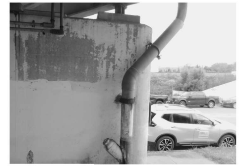
EXIST. DRAINAGE SYSTEM REPAIR: LOCATION 2 - PIER 2 (Looking North)
