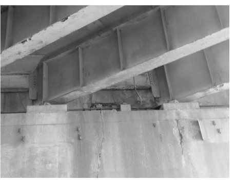
EXISTING ELECTRICAL BOX - NORTH ABUTMENT
