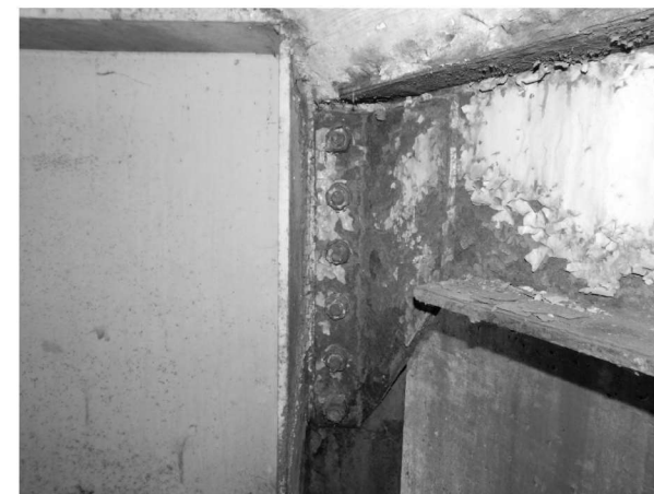
PHOTO 1 - AT BEAM 1B
