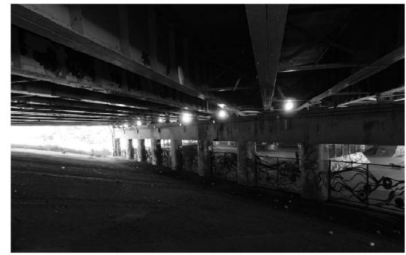
EXISTING LIGHTING: PIER 1 (Looking South)
