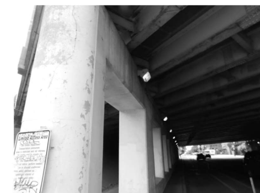
EXIST. LIGHTING: PIER 1 (Looking Southeast)
