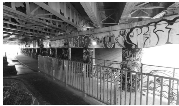
EXISTING LIGHTING: PIER 1 (Looking North)
