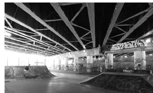
EXISTING LIGHTING: PIER 2 (Looking South)
