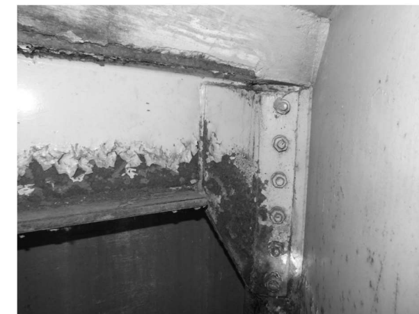
PHOTO 2 - AT BEAM 1A
