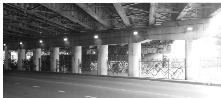
EXISTING LIGHTING: PIER 2 (Looking North)
