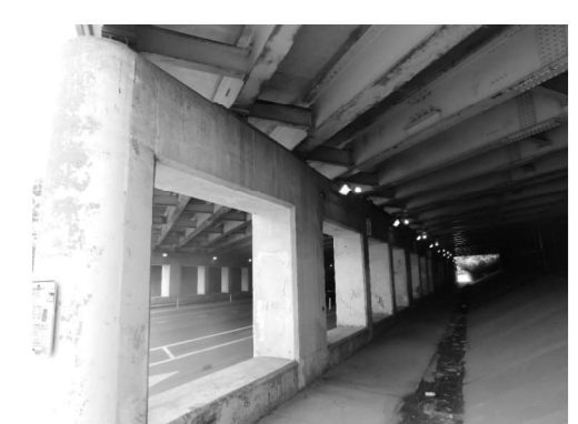
EXIST. LIGHTING: PIER 2 (Looking Southeast)
