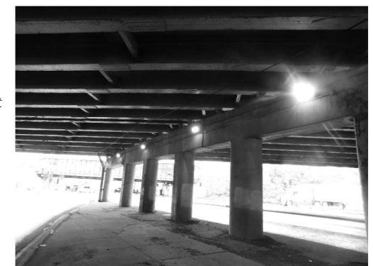
EXISTING LIGHTING: PIER 1 (Looking East)
