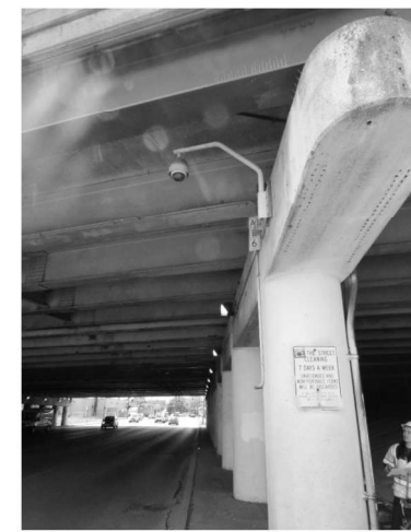
EXISTING LIGHTING: PIER 1 (Looking South)
