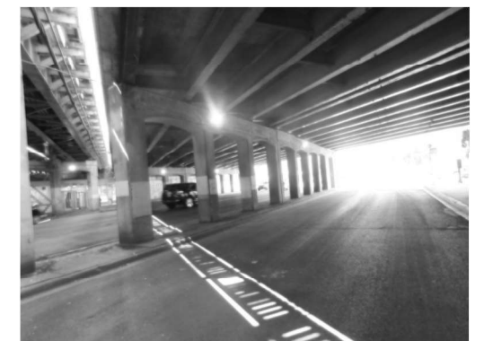
EXISTING LIGHTING: PIER 1
