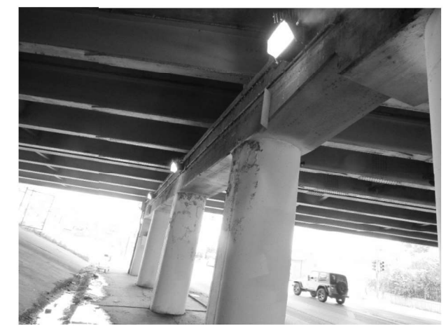
EXISTING LIGHTING: PIER 1 (Looking Northeast)
