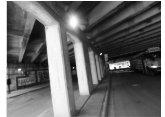
EXISTING LIGHTING: PIER 1
