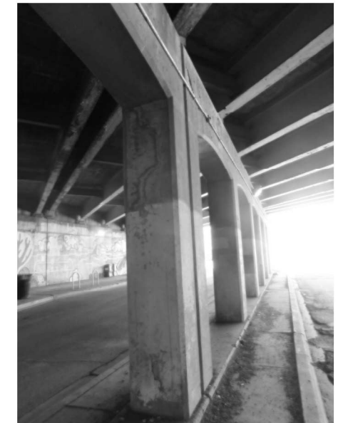
EXISTING LIGHTING: PIER 2 (Looking Northwest)
