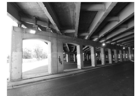
PIER 2 (Looking Southeast)
