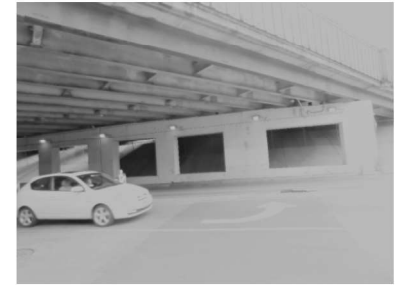
EXISTING LIGHTING: PIER 1 (Looking West)
