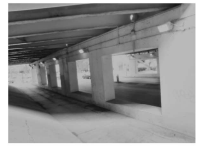
EXISTING LIGHTING: PIER 1 (Looking Northeast)
