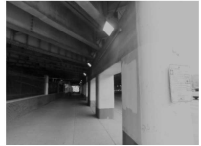
EXISTING LIGHTING: PIER 2 (Looking Northwest)
