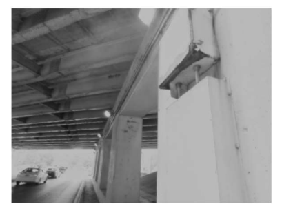
EXISTING LIGHTING: PIER 2 (Looking North)
