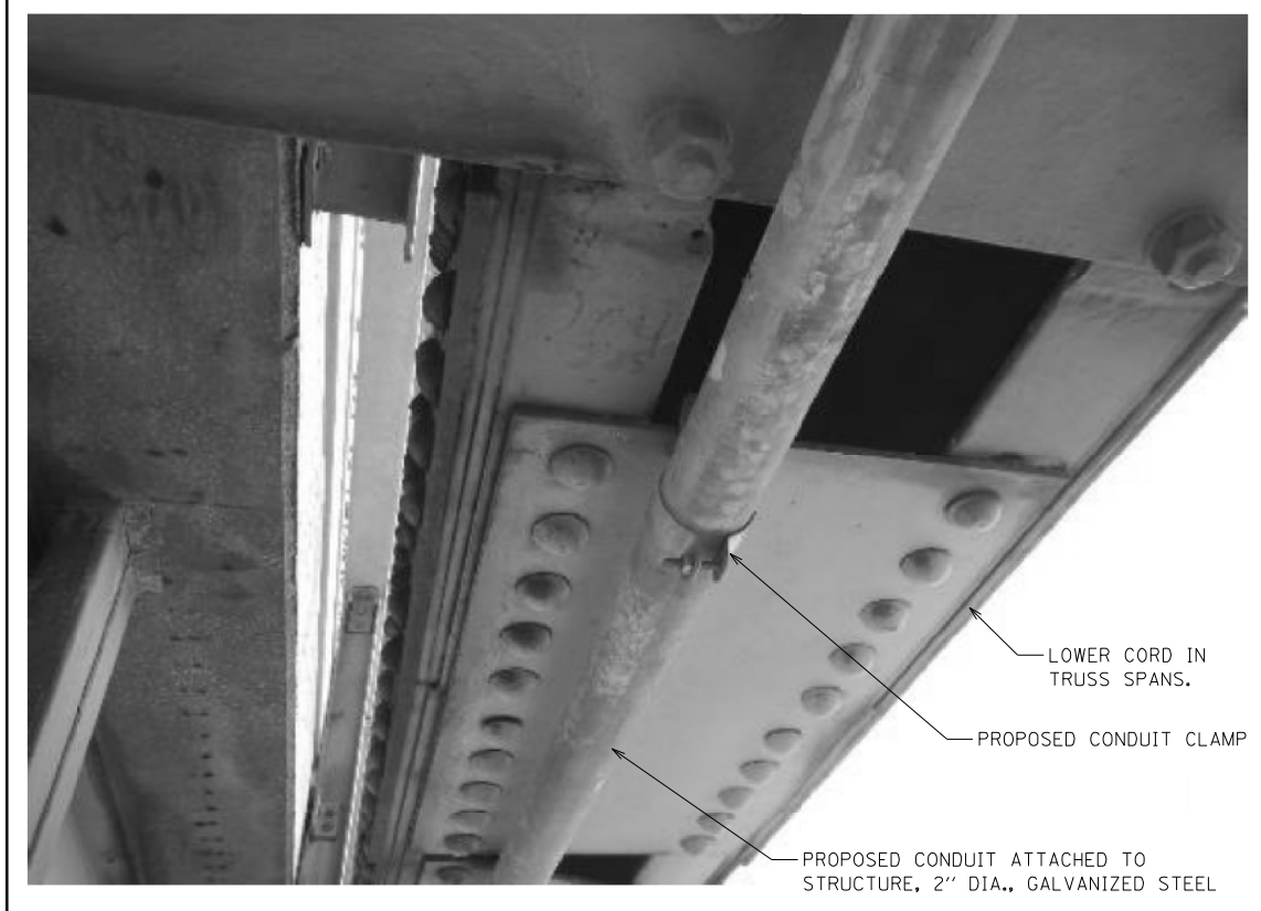
CONDUIT ATTACHED TO STRUCTURE DETAIL
