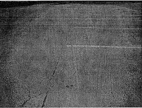
Photograph 9: Facing south in southwestern parking area, moderate severity joint separation with spalled interconnected cracks.
