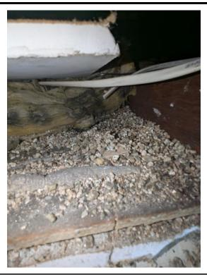
**Material Description:** Vermiculite Insulation - Tested Positive for Asbestos
