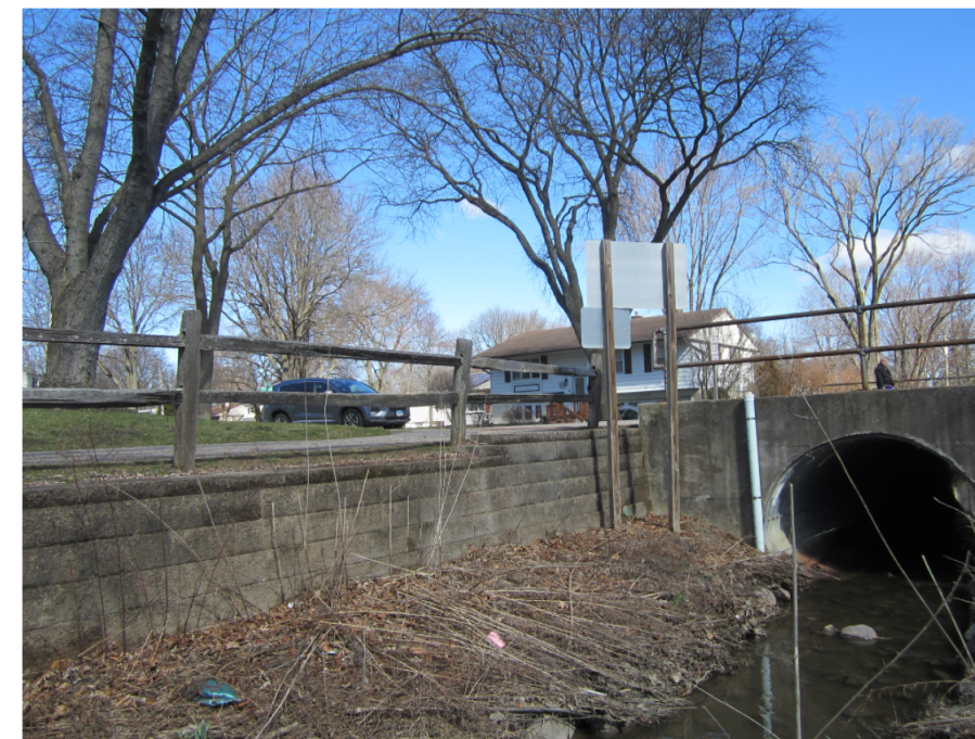
PHOTO - REMOVE AND RE-ERECT SEGMENTAL BLOCK WALL
