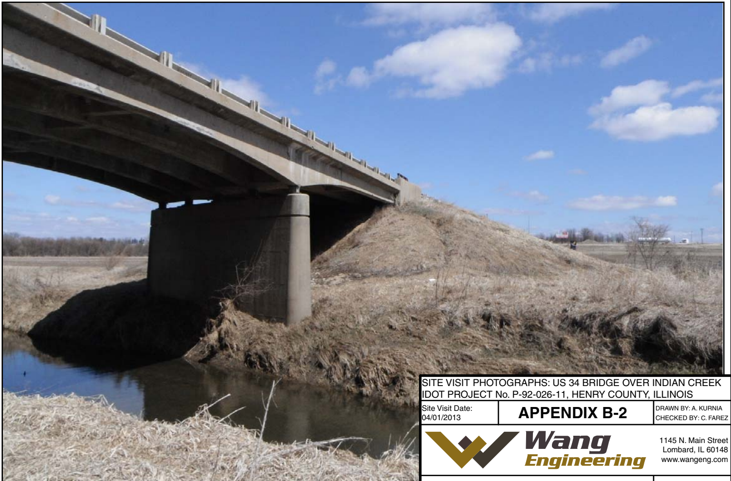
Existing Pier 2 and East Abutment
