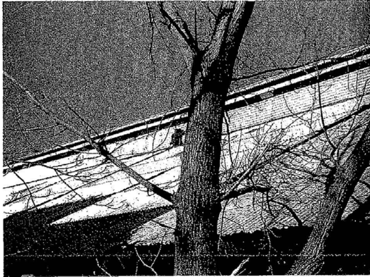
Transite Building - Roof
