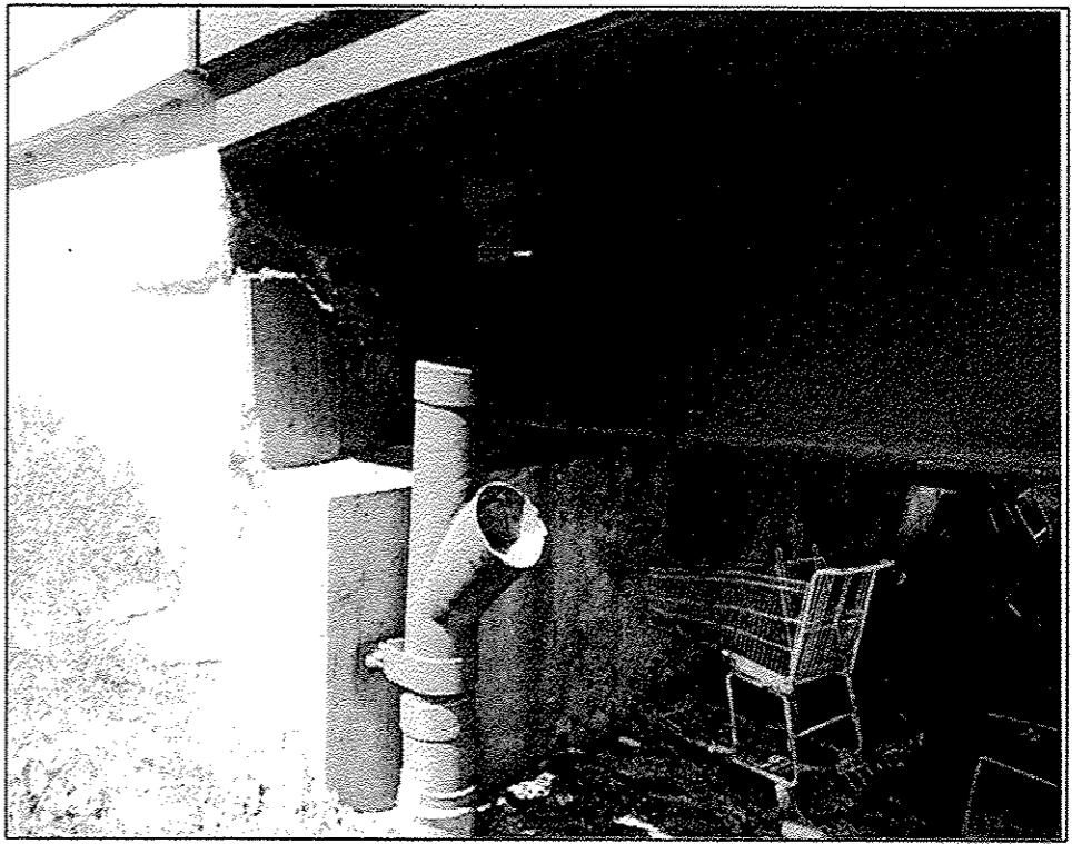
016-1140 PHOTO #1 P18 (ABUTMENT)
