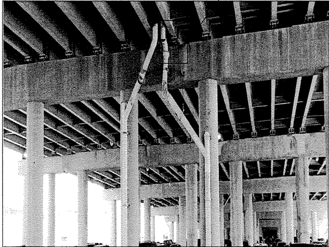
016-0137 - PHOTO #1 SOUTH FACE OF PIER 11
