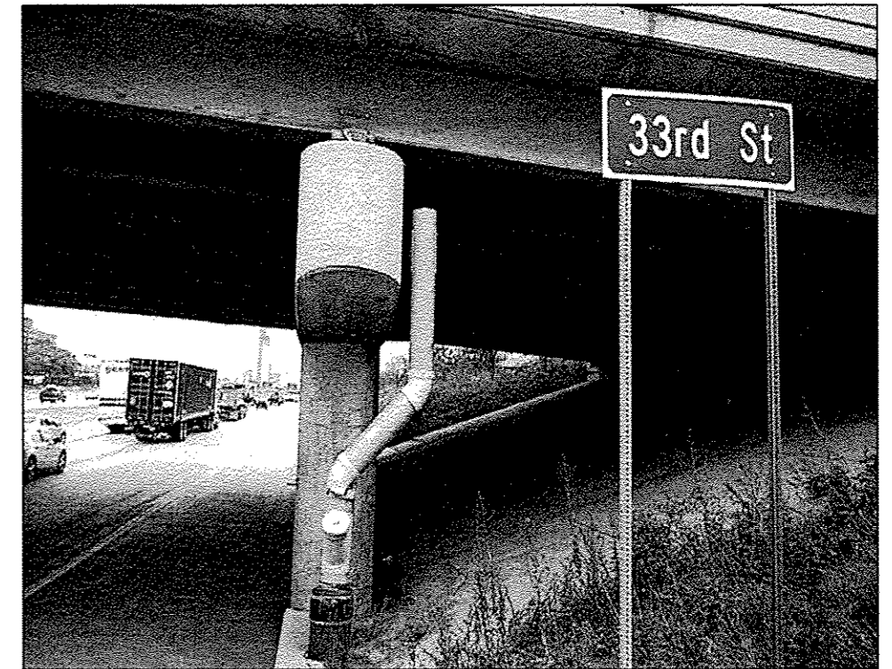
016-1158 PHOTO # PIER 6 _ SOUTH END
