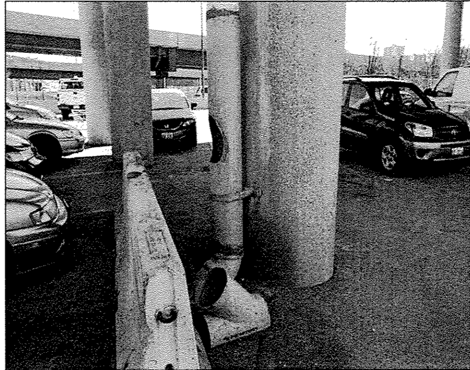
016-1067 PHOTO #2 PIER A6
