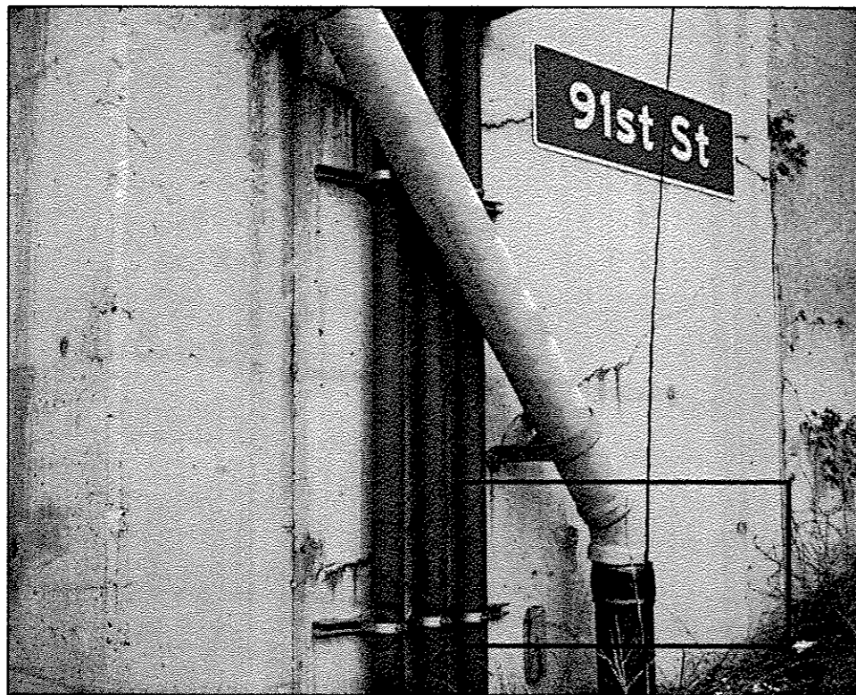
016-1141 PHOTO #3 EAST ABUTMENT _ SOUTH END
