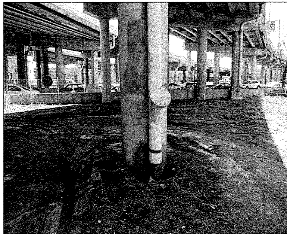
016-1067 PHOTO #5 SPAN A15
