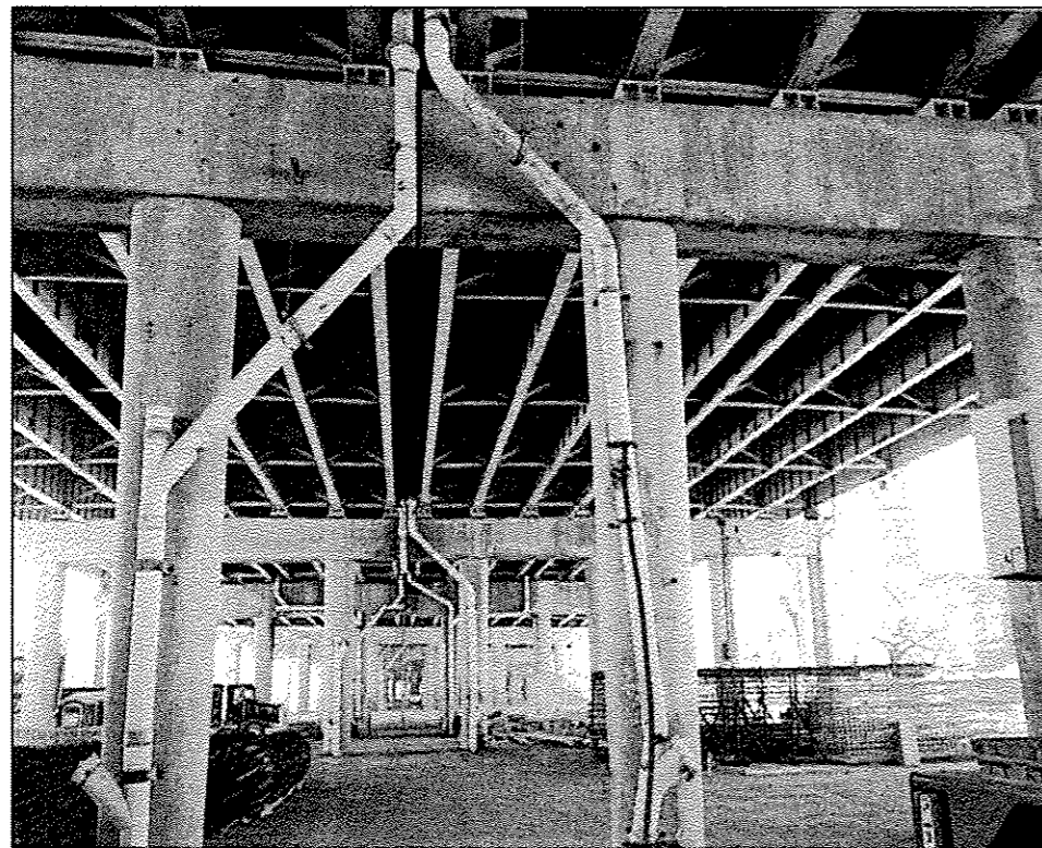
016-1111 PHOTO #4 MAIN LINE PIER 4 _ NORTH FACE
