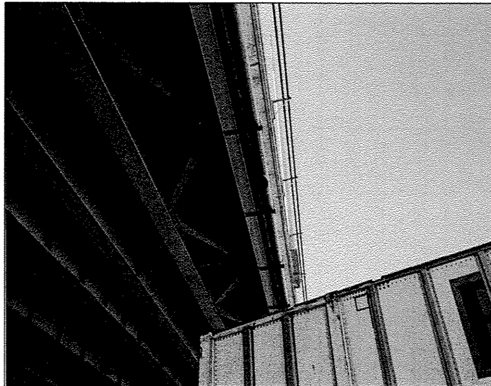
016-1116 PHOTO #2 NORTH FASCIA BEAM - MID SPAN 2
