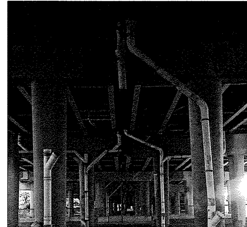
016-1111 PHOTO #3 MAIN LINE PIER 3 _ NORTH FACE
