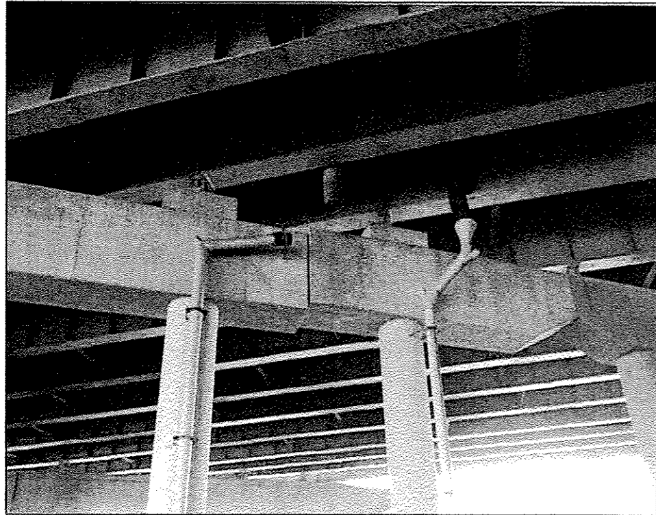
016-0004 AND 016-0005 PHOTO #1 PIER 2 _ WEST FACE
