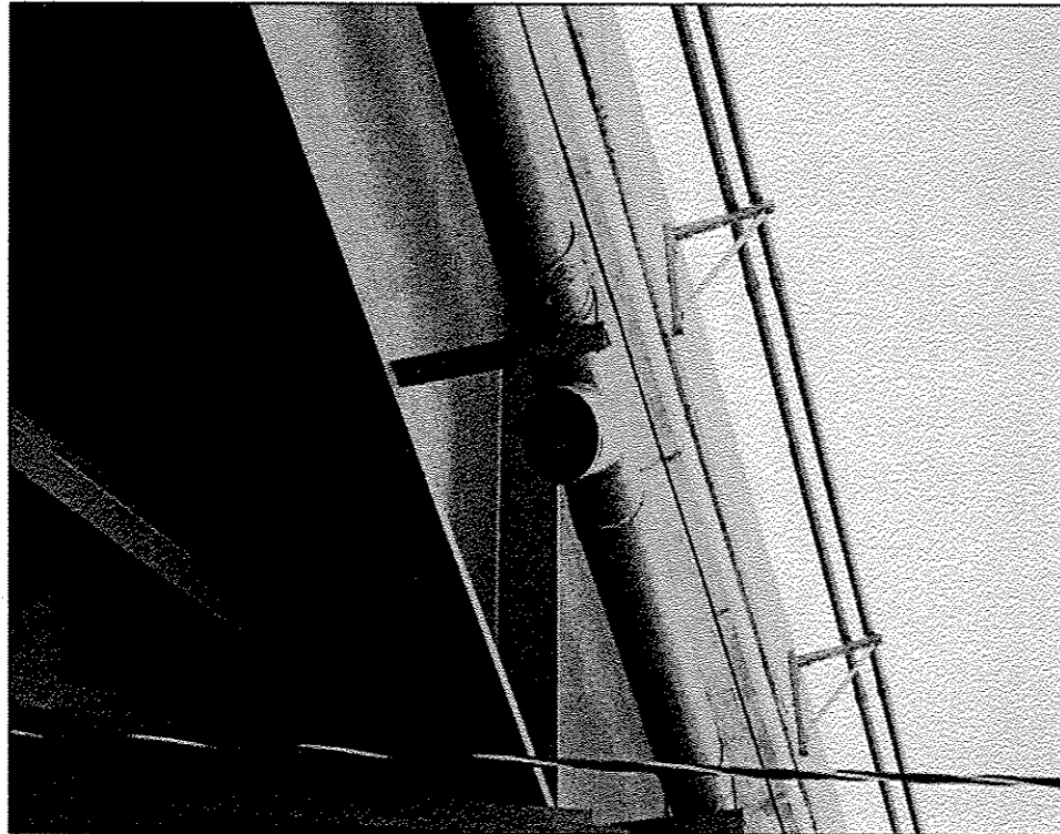
016-1116 PHOTO #1 NORTH FASCIA BEAM SPAN 2 - WEST OF PIER 2
