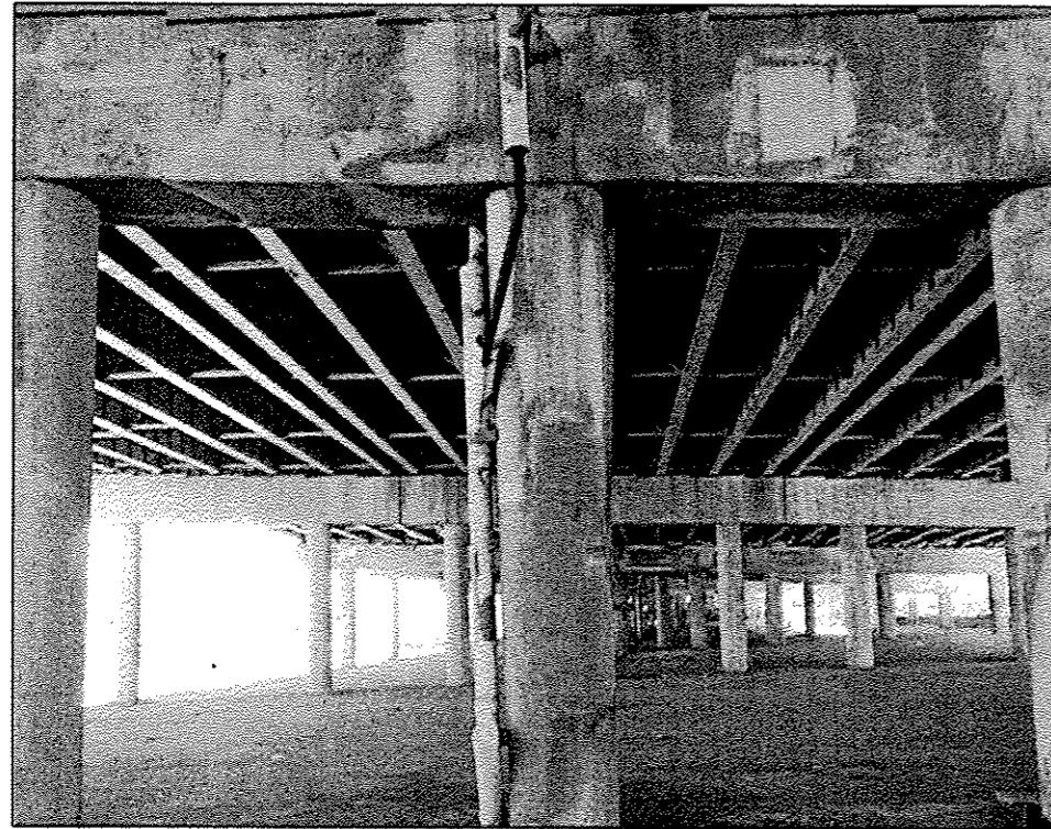
016-1112 PHOTO #1 MAIN LINE PIER 30 _ NORTH FACE
