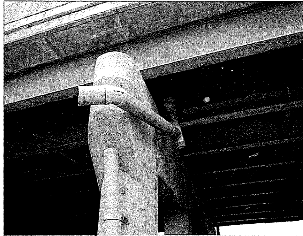
016-1151 PHOTO #2 PIER 1 _ SOUTH END
