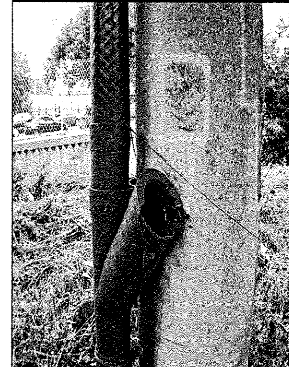
016-1047 PHOTO #2 PIER 27 - CLOSE UP
