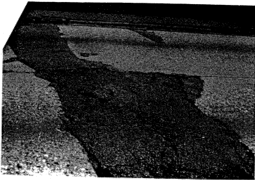
High Severity Asphalt Patch Deterioration
